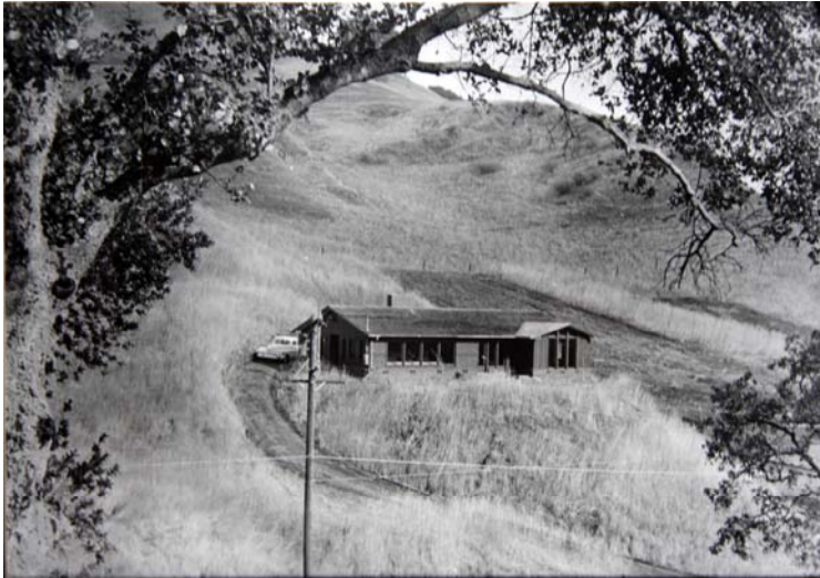
The Paterson House under construction circa 1950 photo courtesy of Dorothee Paterson
