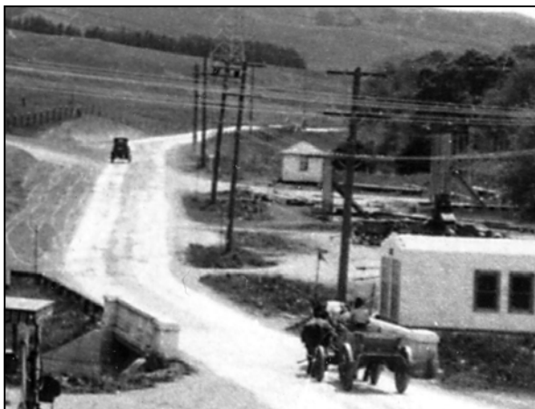
San Pablo Creek Bridge in 1924 looking toward Orinda Village from Camino Pablo
